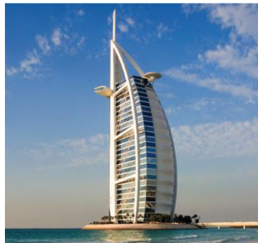
Figure 3: Tertiary Sector – The Breathtaking Burj Al Arab Hotel in Dubai 3
